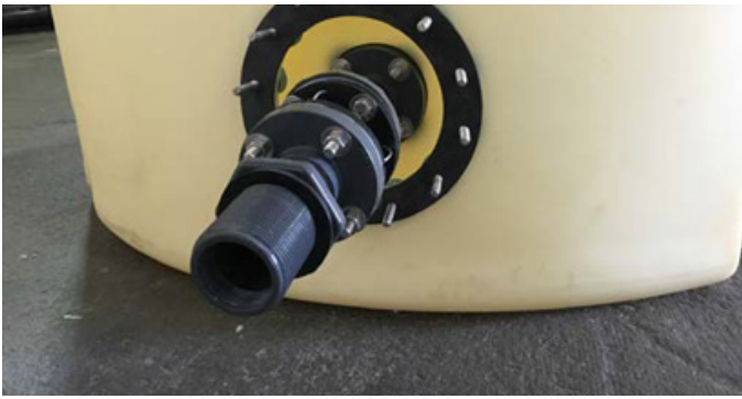
INSTALL 8" GASKET ON OUTER TANK
